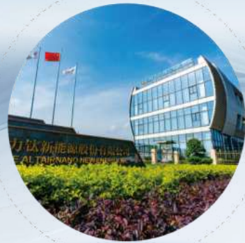
Zhuhai Industrial Park (headquarter)
